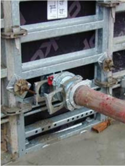
Fig. 3. Pouring in formwork
