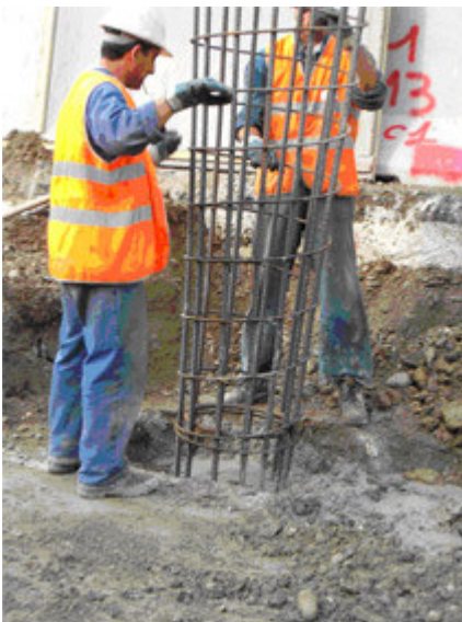
Fig. 5. Easy cage fitting for drilled foundation piles
